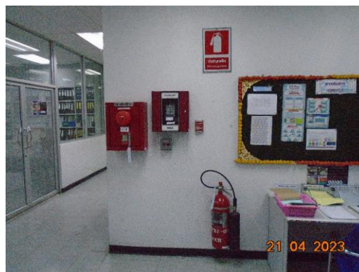
Manual Fire Alarm & Fire Extinguisher
